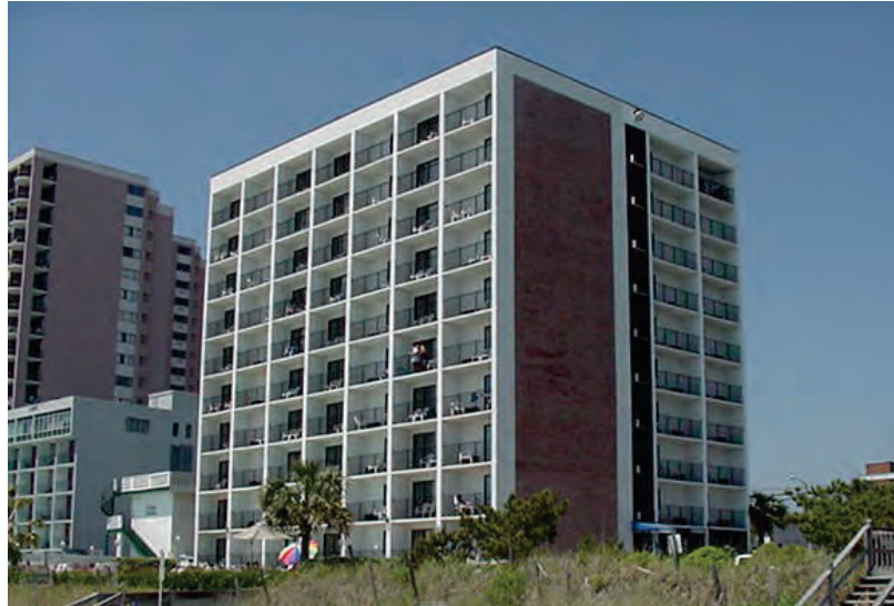
Figure 3-5 Typical reinforced masonry multi-family residential building (photo credit: G. Kingsley).
