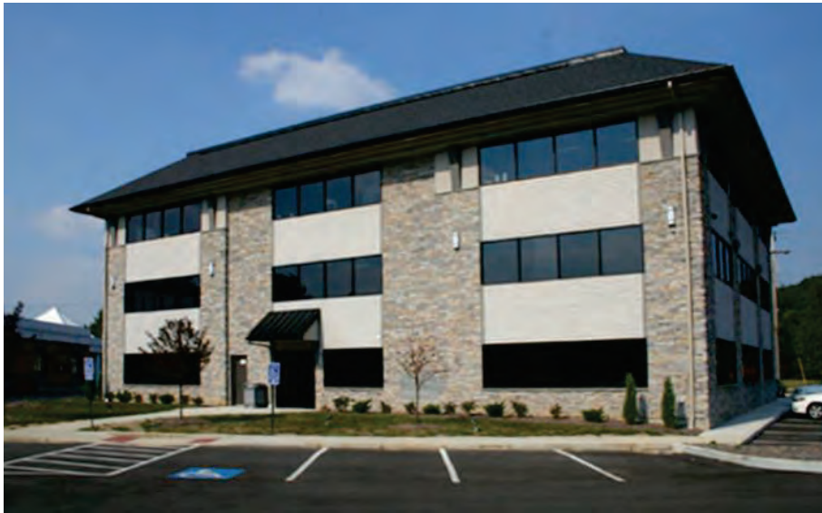
Figure 3-4 Typical reinforced masonry commercial office building (photo credit: FEMA P-749, Chapter 4, Figure 23).
